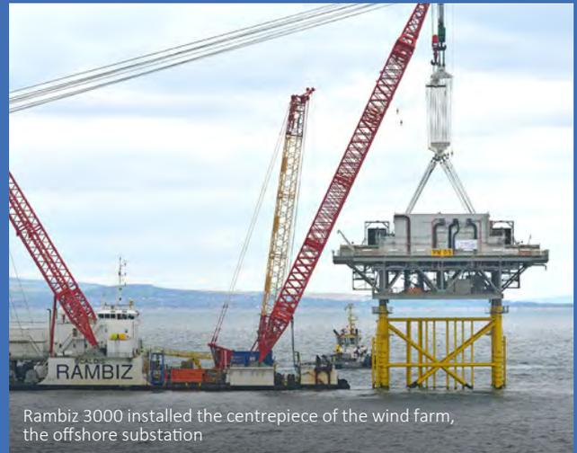
Rambiz 3000 installed the centrepiece of the wind farm, the offshore substation
